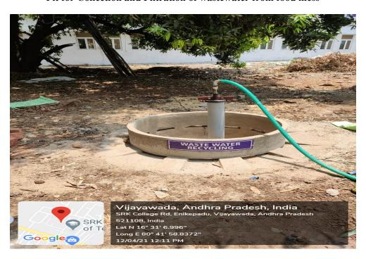
Filtered water collected into a Bore well and lifted using 1 HP Pump
